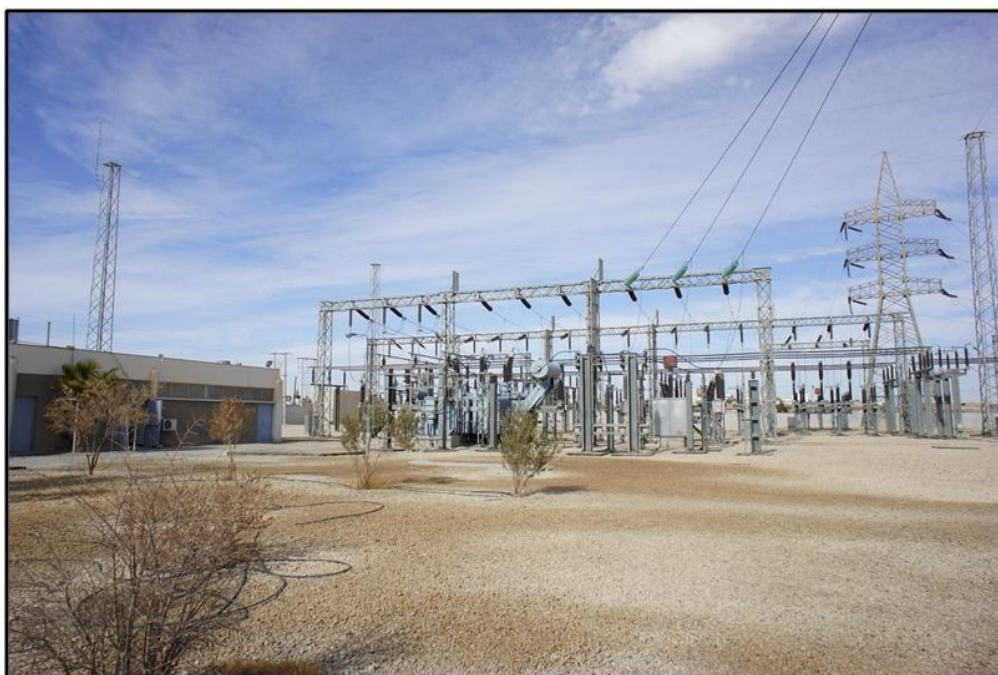
Figure 3-6: Typical 33/220kV Substation
