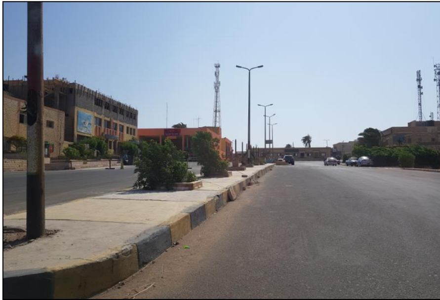
Figure 8-65: Zaafarana--Ras Gharib Road
