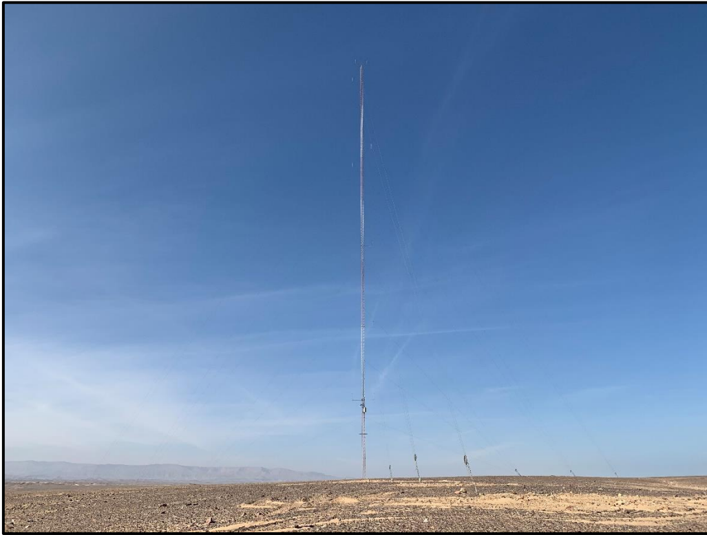
Figure 8-62: Met Mast Located Onsite
