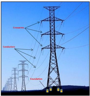
**Figure 6: Typical Structural Components of towers**
