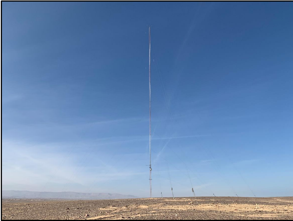
Figure 8-63: Met Mast Located Onsite
