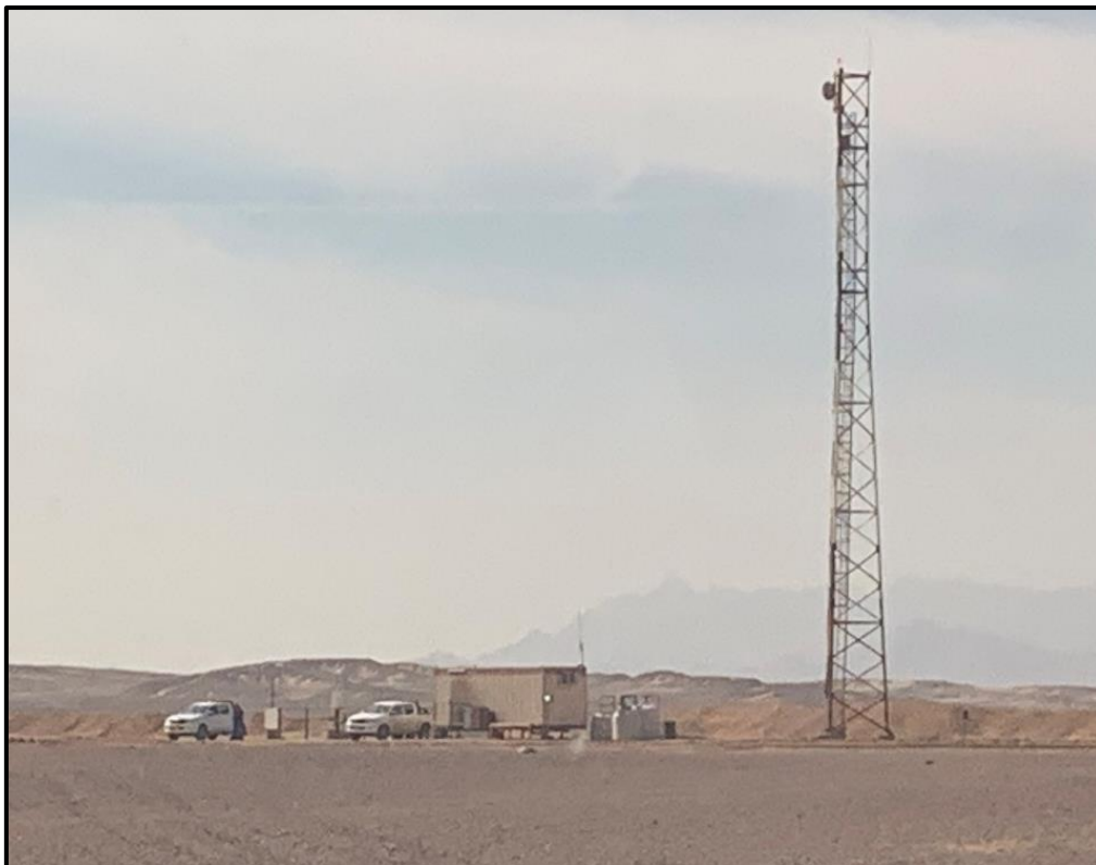
Figure 8-62: Telecommunication Tower within Petroleum Storage Facility Onsite
