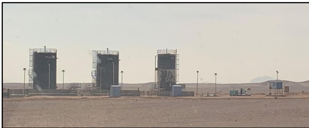
Figure 8-8: Petroleum Storage Facility
