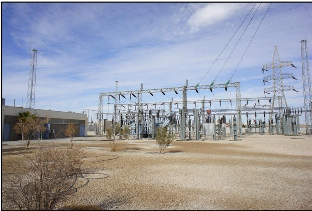
Figure 3-6: Typical 33/220kV Substation
